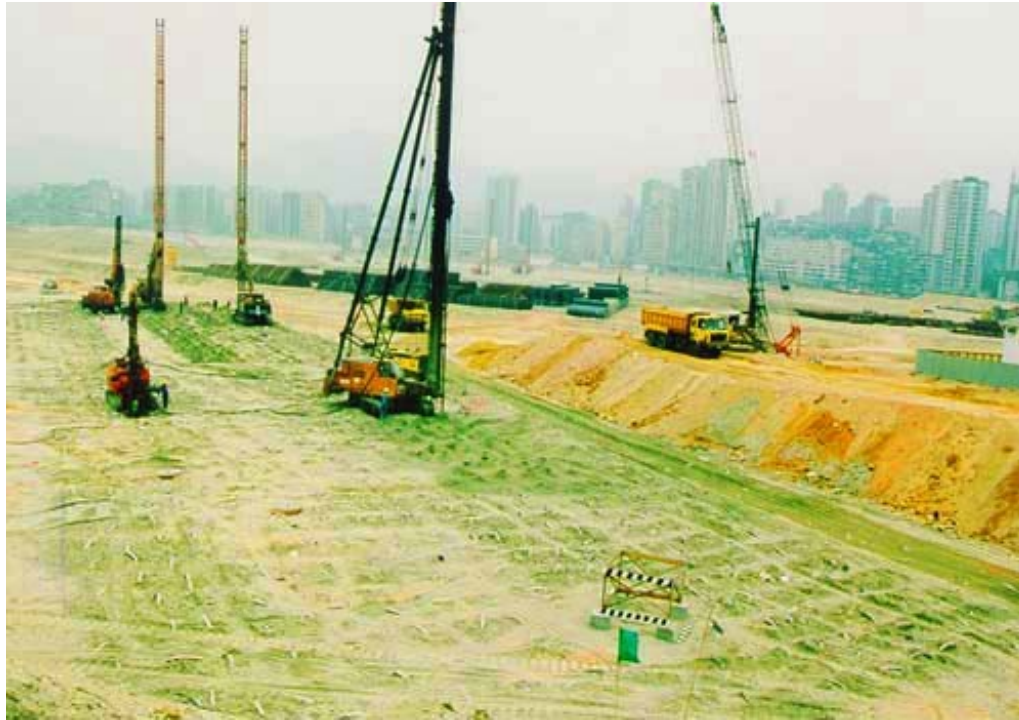
Installation of PVDs
